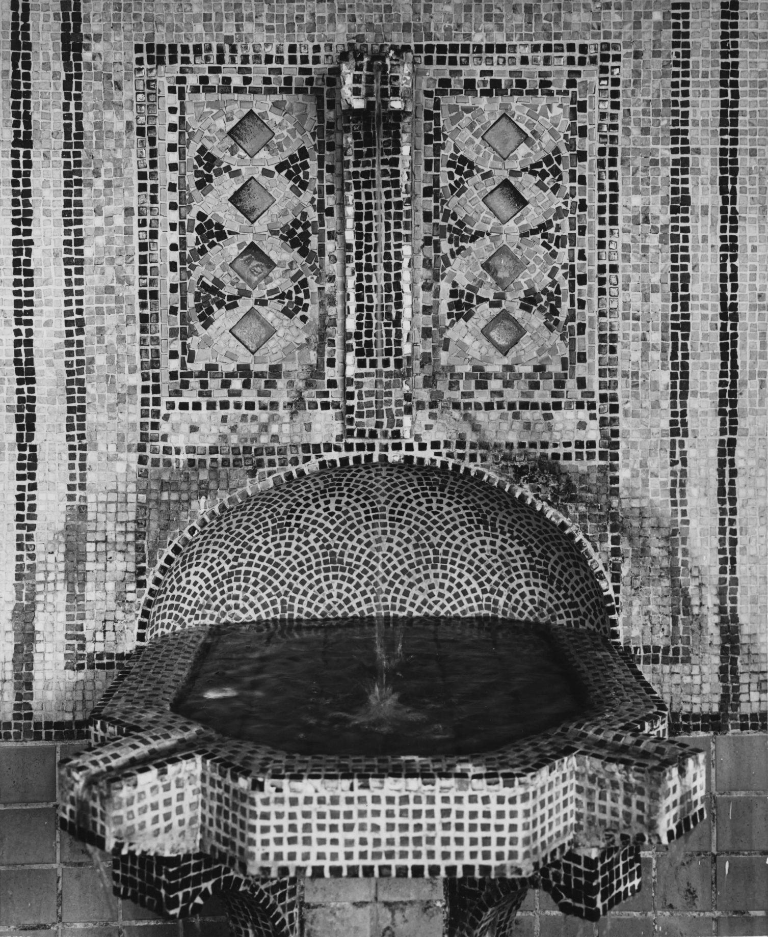
2. Dodge House Irving Gill, Architect North End of Formal Garden
