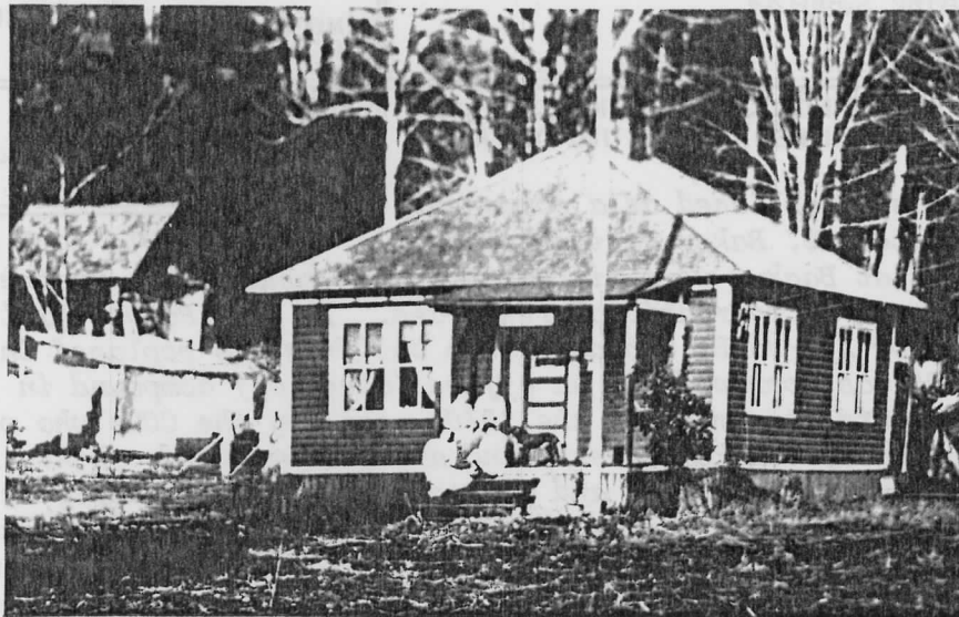
BACKUS RANGER STATION, PRE-1916 (photo. by N. Hicks)
