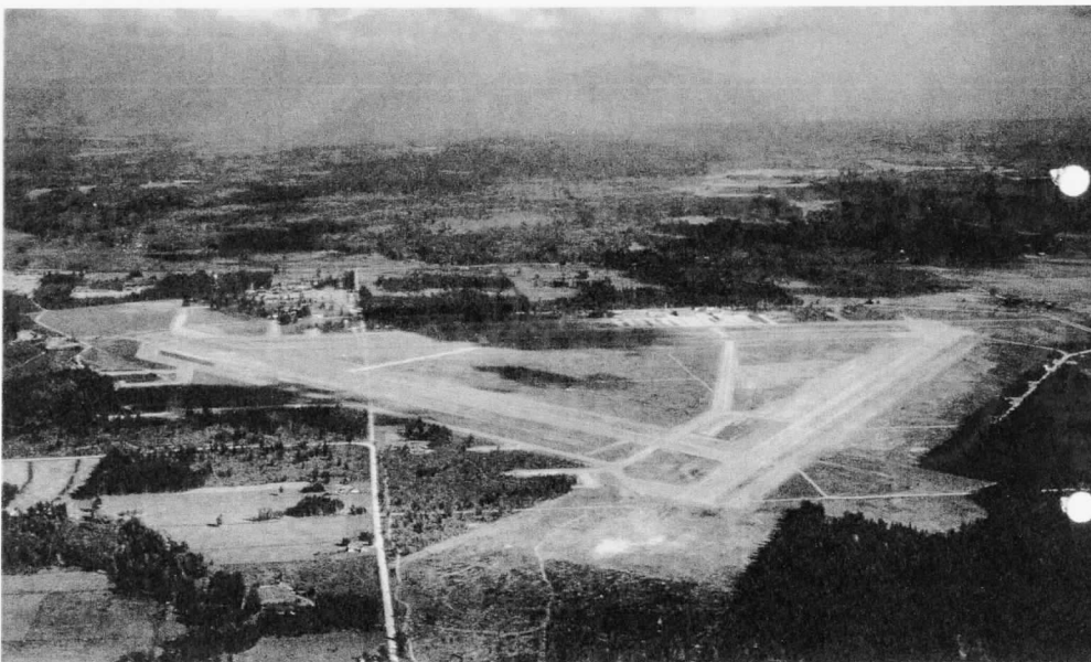
Extensive improvements to both the field and building area at U.S. Naval Auxiliary Air Station, Arlington, are visible in the photograph, dated 25 Dec. 1945. Contrasting with photograph of 19 Oct. 1943, note completion of third runway at right and development of Ground Training and Class "C" overhaul facilities behind hangar, center right. New fire house is discernible at center right, and extensive new Public Works facilities in main station area, upper left. SOURCE: National Archives & Records Administration, Seattle Branch Record Group 181, Wartime Histories of Units.
