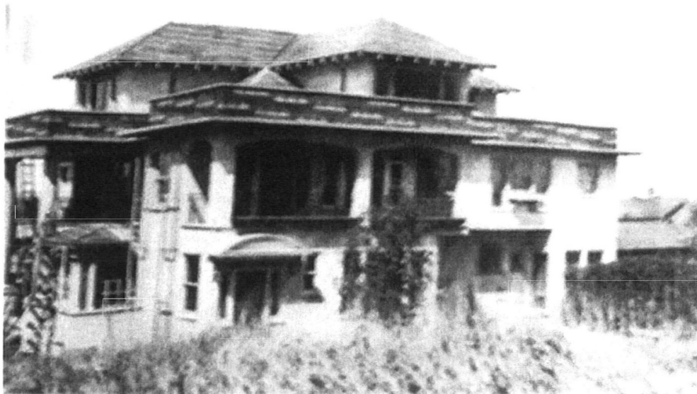
Axtell House after conversion to apartments showing extension of portico, additional wing, stucco treatment, modernized roof and windows created for Frances Axtell's conversion of her home into apartments. c. 1926. Photograph courtesy of William B. Hussey.
