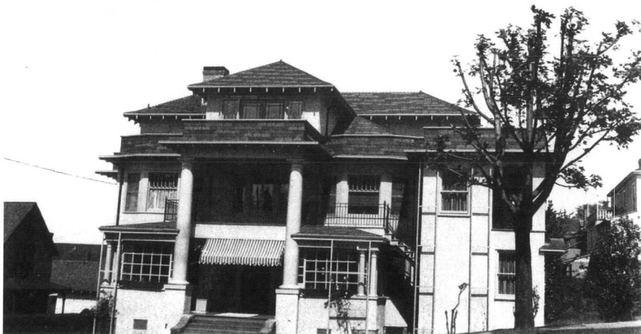
Axtell Apartments showing extension of portico, additional wing, stucco treatment, modernized roof and windows created for Frances Axtell's conversion of her home into apartments. c. 1927. Photograph courtesy of William B. Hussey.
