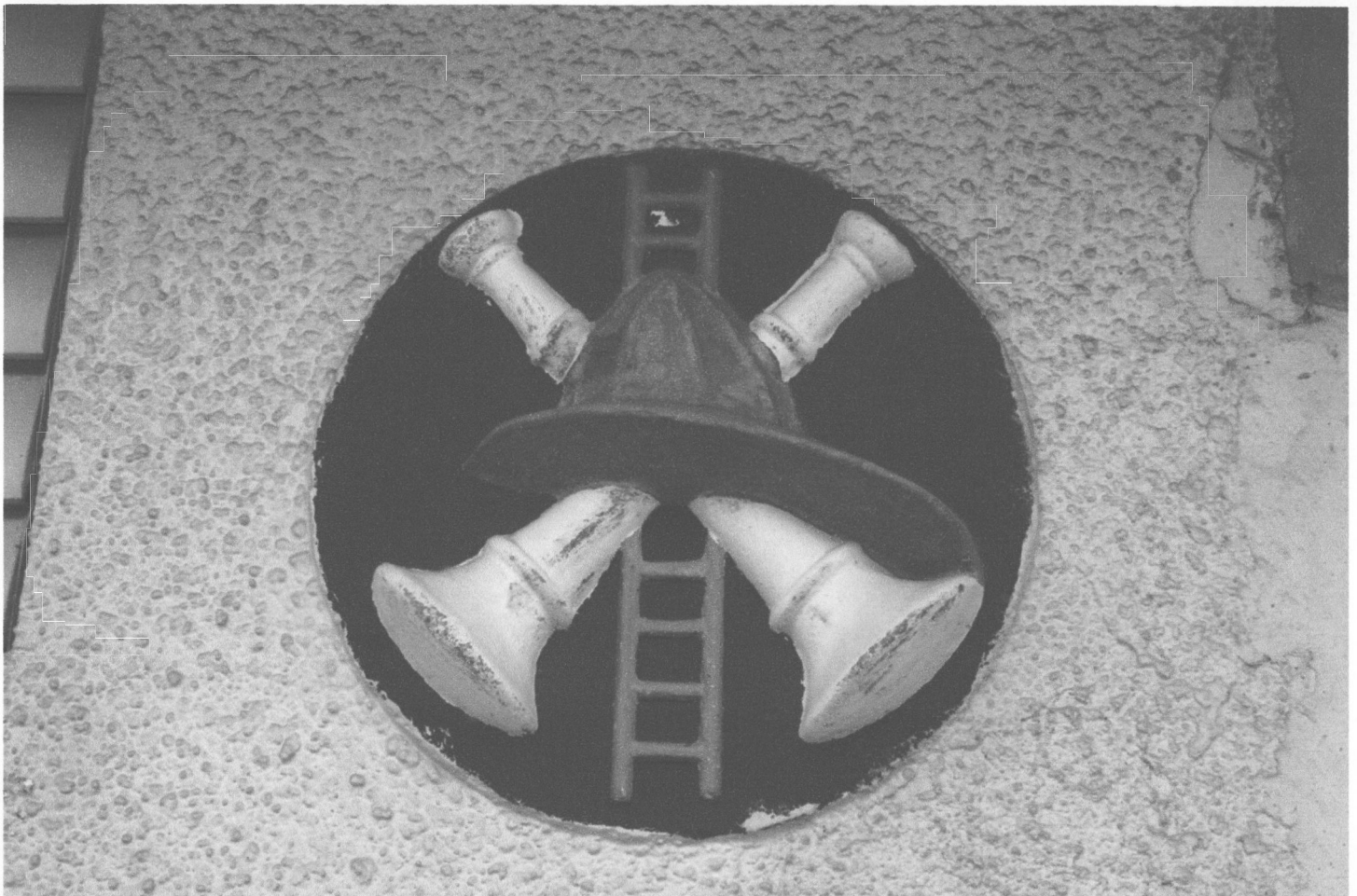
Fig. 10: Escutcheon incorporates the fireman's distinguishing symbols: the hat, ladder and blow horns. Photo: Jorge Rigau, 2011
