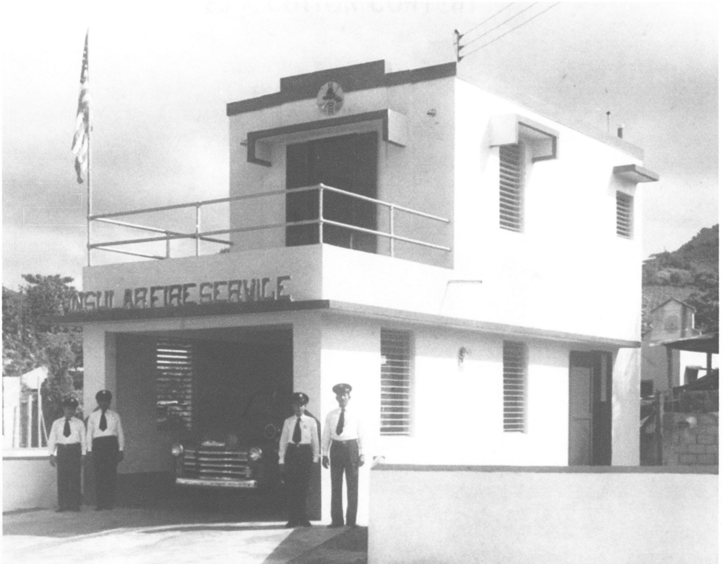
Fig. 23: Prototype A at an unidentified location. Source: Cuerpo de Bomberos de Puerto Rico
