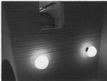
Fig. 4 Tongue and groove wood plank bell tower ceiling
