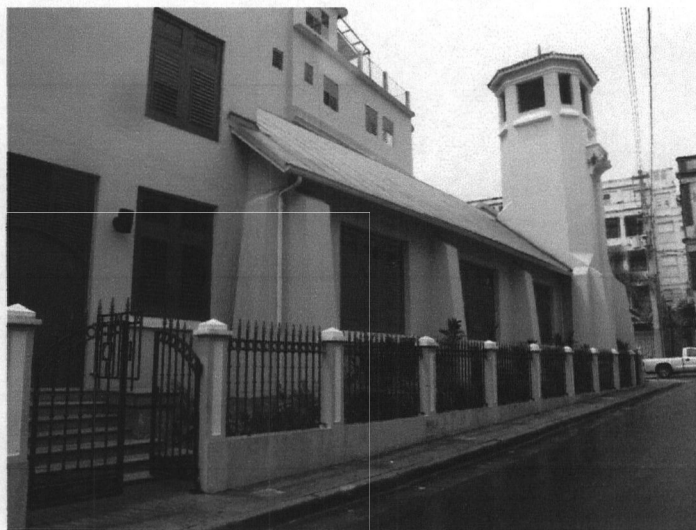
Fig. 10 Buttress on the West façade
