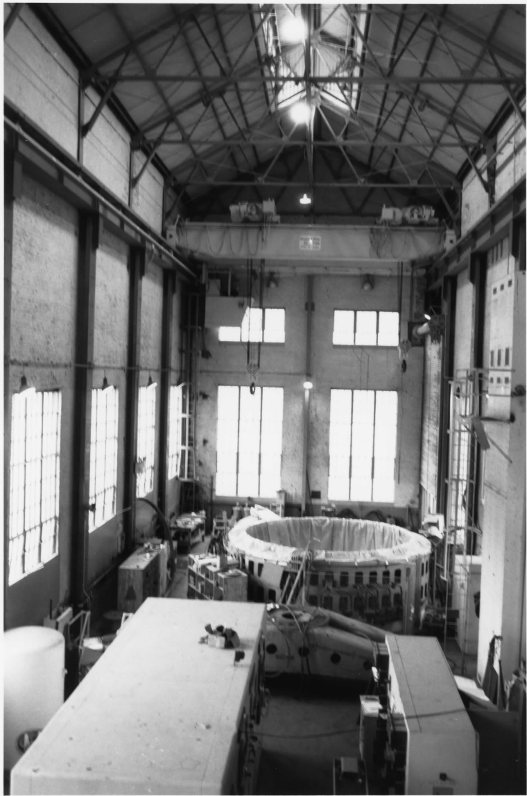
Great Falls Hydroelectric Station Rock Island vicinity, White & Warren Cos., TN # 5 of 6
