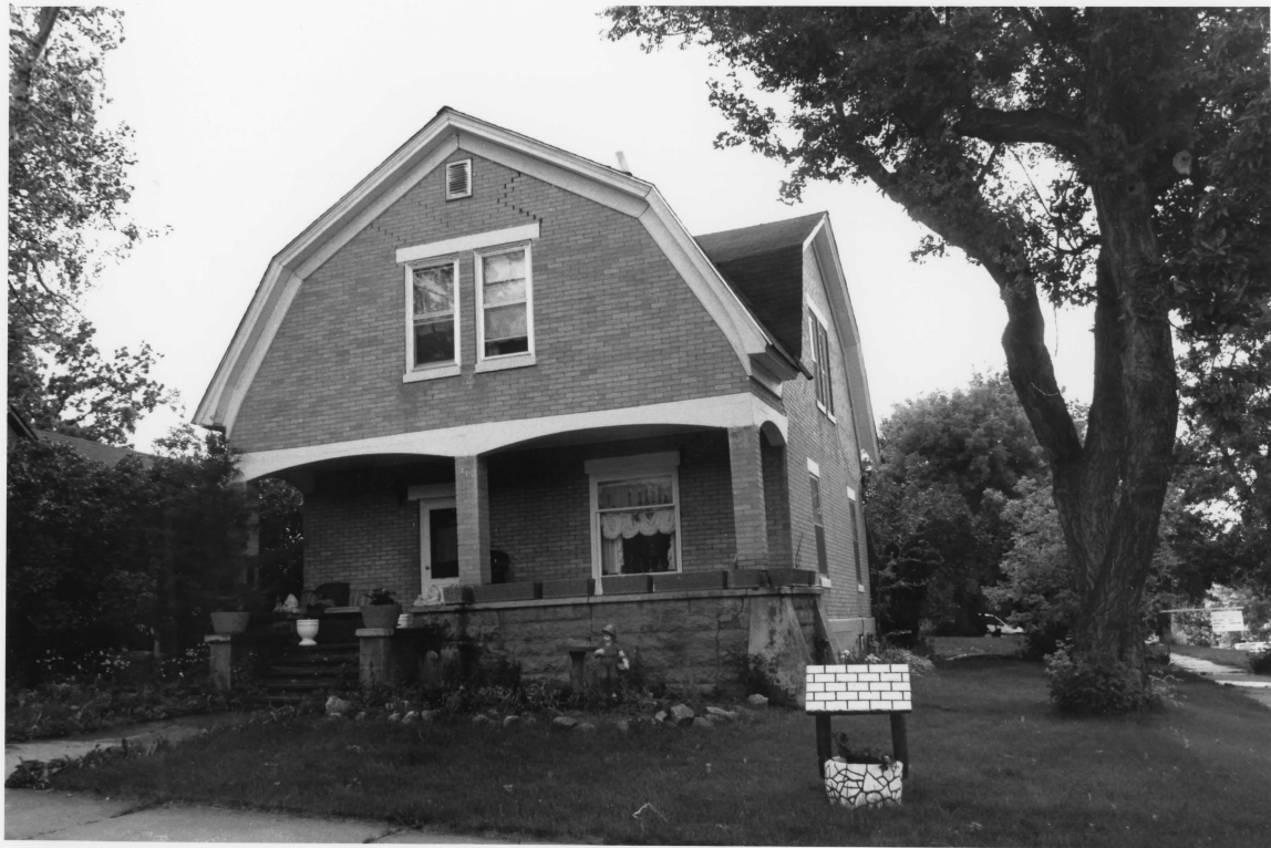
JAMES A CORBIN HOUSE, LAWRENCE CO., S.D. No 1
