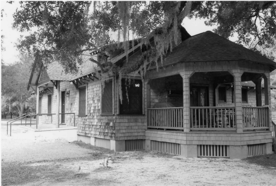
22. Gravel Hill Plantation 3954 Augusta Stage Coach Road, Garnett vicinity Hampton County, South Carolina
