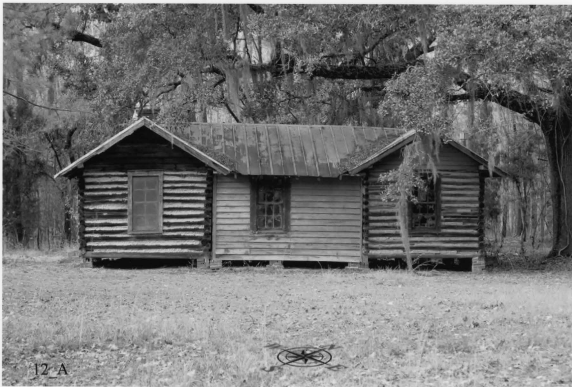
34. Gravel Hill Plantation 3954 Augusta Stage Coach Road, Garnett vicinity Hampton County, South Carolina
