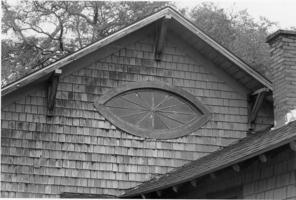
29. Gravel Hill Plantation 3954 Augusta Stage Coach Road, Garnett vicinity Hampton County, South Carolina
