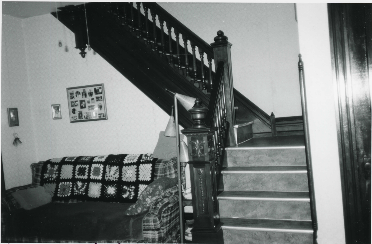
Bayer Angstadt Farm Berks Co., Pa. Parlor - 1905 house east view
