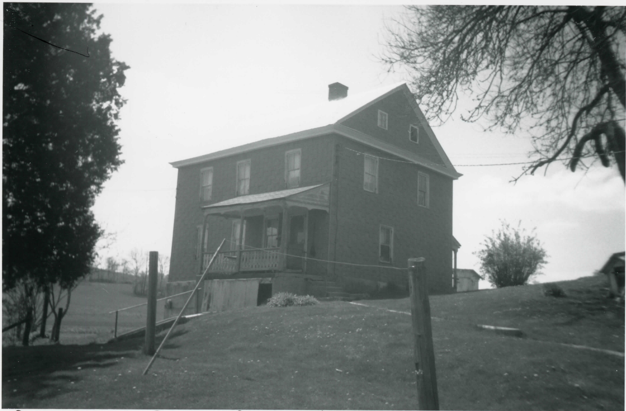
OXENRIDER FARM, BERKS COUNTY, PA FARM HOUSE, NORTH EAST FACADE
