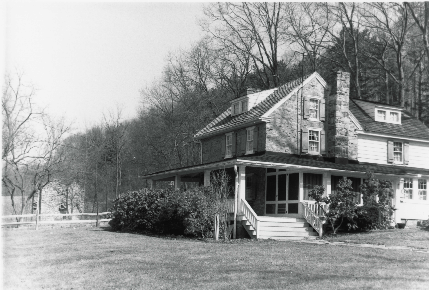
DALEFURNACE AND FORGE HISTORIC DISTRICT, PA PHOTO # E WORKER'S HOUSE AND RUIN OF WORKER'S HOUSE R 41-22 PHOTOGRAPHER: DIANE B. REED - PITMC/BHA 3/8/90
