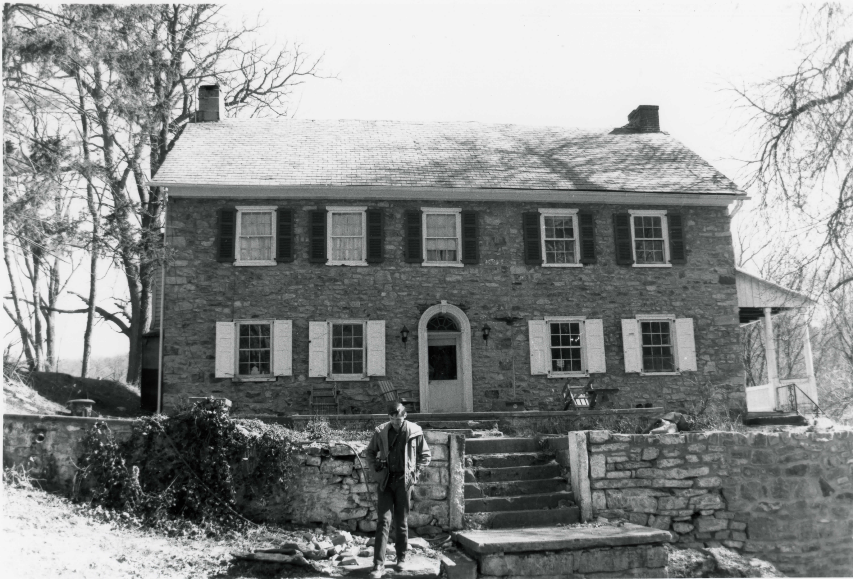
DALE FURNACE AND FORGE HISTORIC DISTRICT, PA PHOTO # A IRONMASTER'S MANSION R41-5 PHOTOGRAPHER: DUANE B. REED - PHMC/BHP 3/8/90
