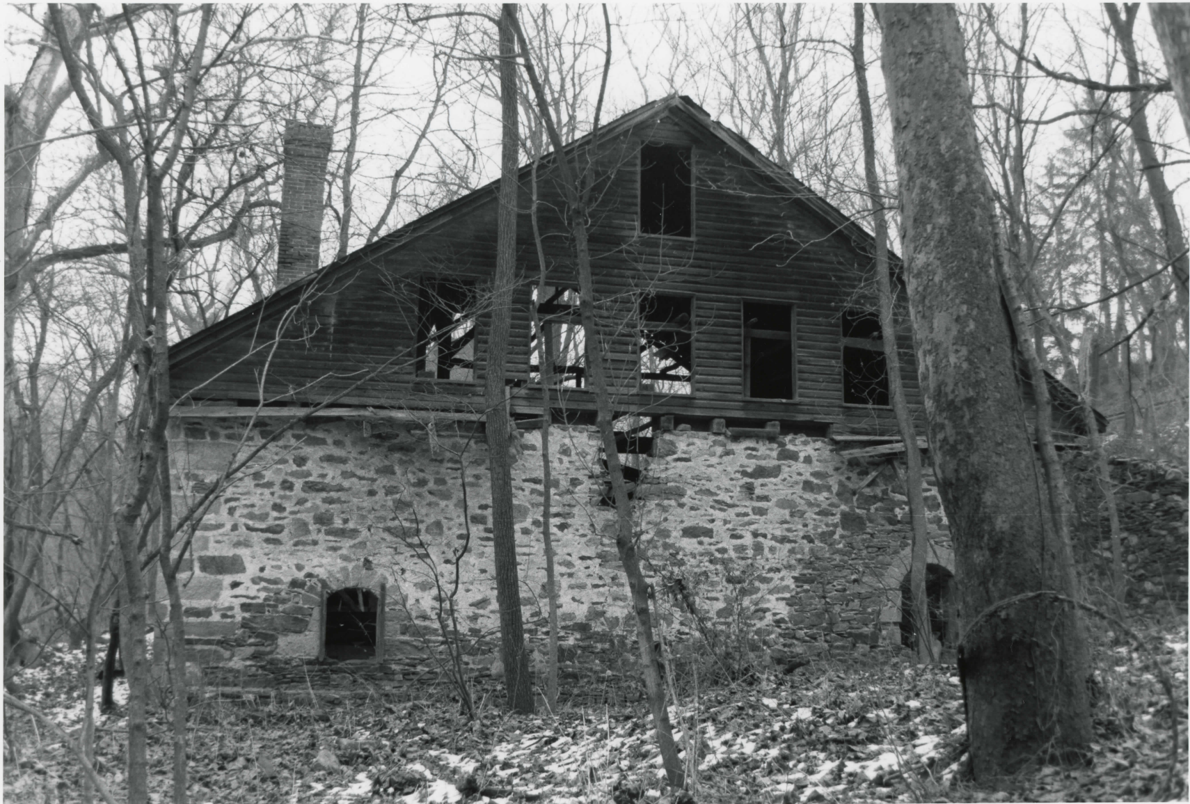
CODORUS FORGE AND FURNACE HISTORIC DISTRICT, PA PHOTO #E FORGE
