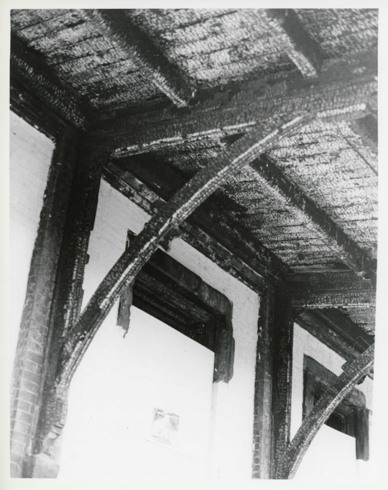
VIEW OF TWO FIRE DAMAGED OVERHANGING ROOF ARCHES AND ABOVE ROOF.
