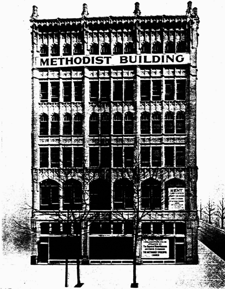
METHODIST BUILDING, 17th and Arch Streets, Philadelphia Ballinger & Perrot, Architects
