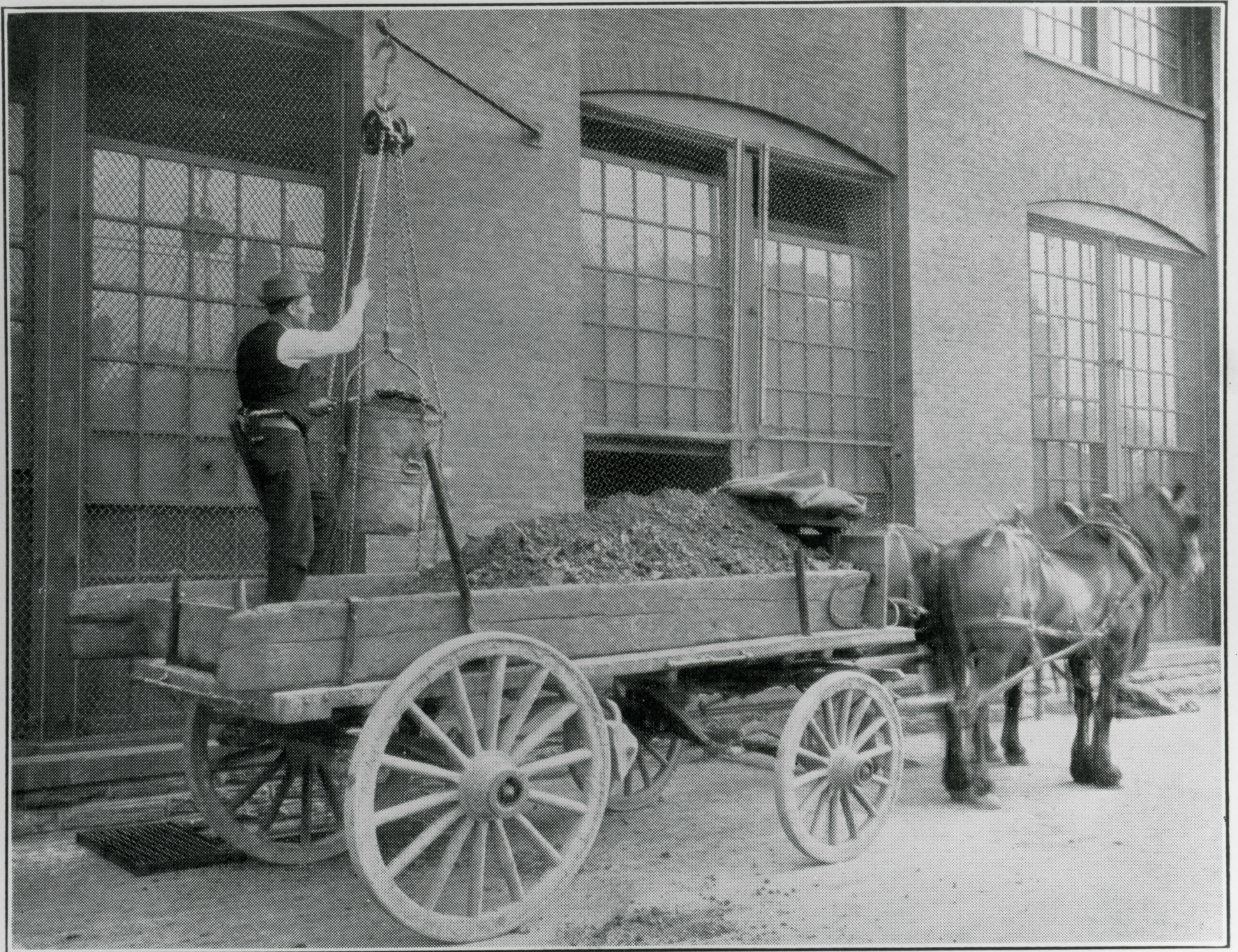
LIFTING ASHES FROM BASEMENT WITH QUICK SPEED PEERLESS HOIST
