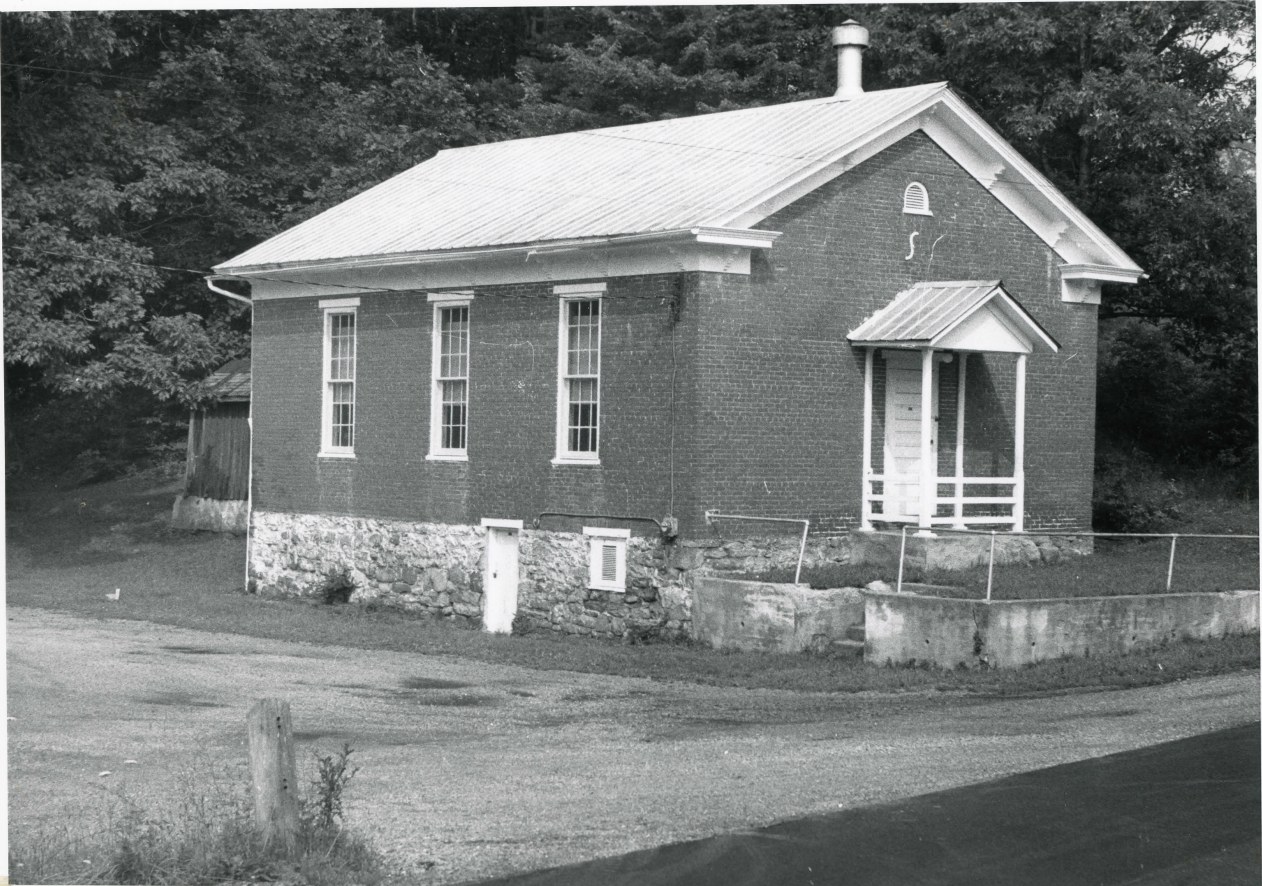
VIEW OF SCHOOL HOUSE TAKEN FROM CENTER OF ROAD LEADING FROM U.S. RTE 522 TO VIRA, PA.
