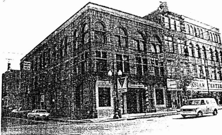
Pittsburgh National Bank at the corner of Penn and Wood. Formerly First National Bank of Wilkesburg founded in 1892.
