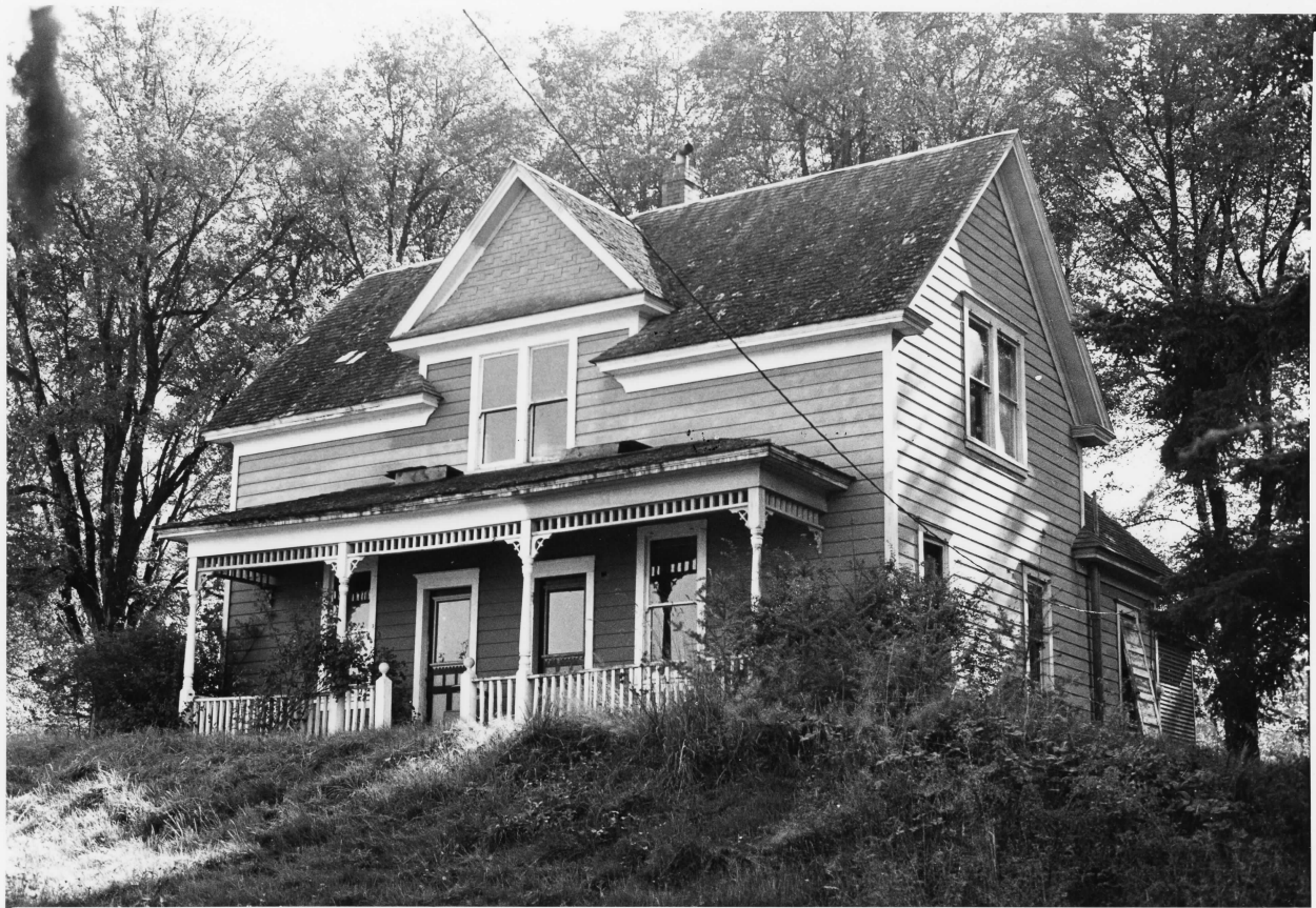
ORIGINAL FARM HOUSE
