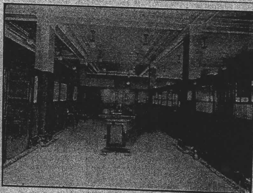
THE FIRST NATIONAL'S NEW BANKING ROOM
