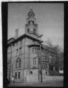
South and east facade Looking northwest
