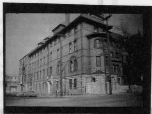
South facade, Looking Northwest
