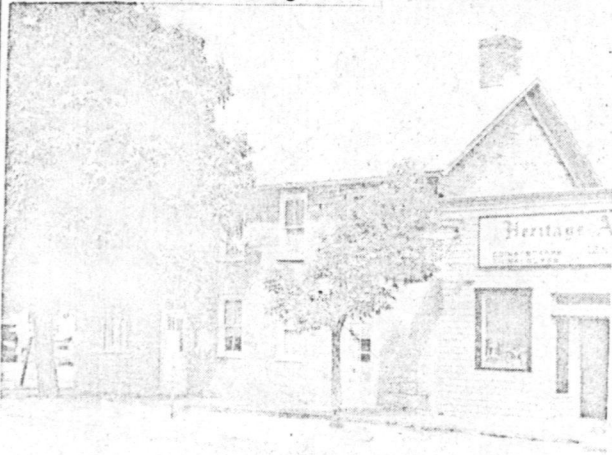
Thomas House, 6 S. High St., Dublin
