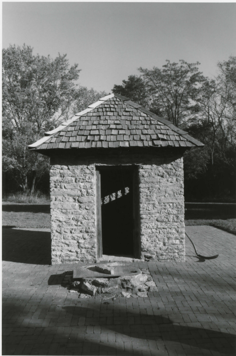
Harmony Hill Dairy House, Clermont Co., OH Photo 5
