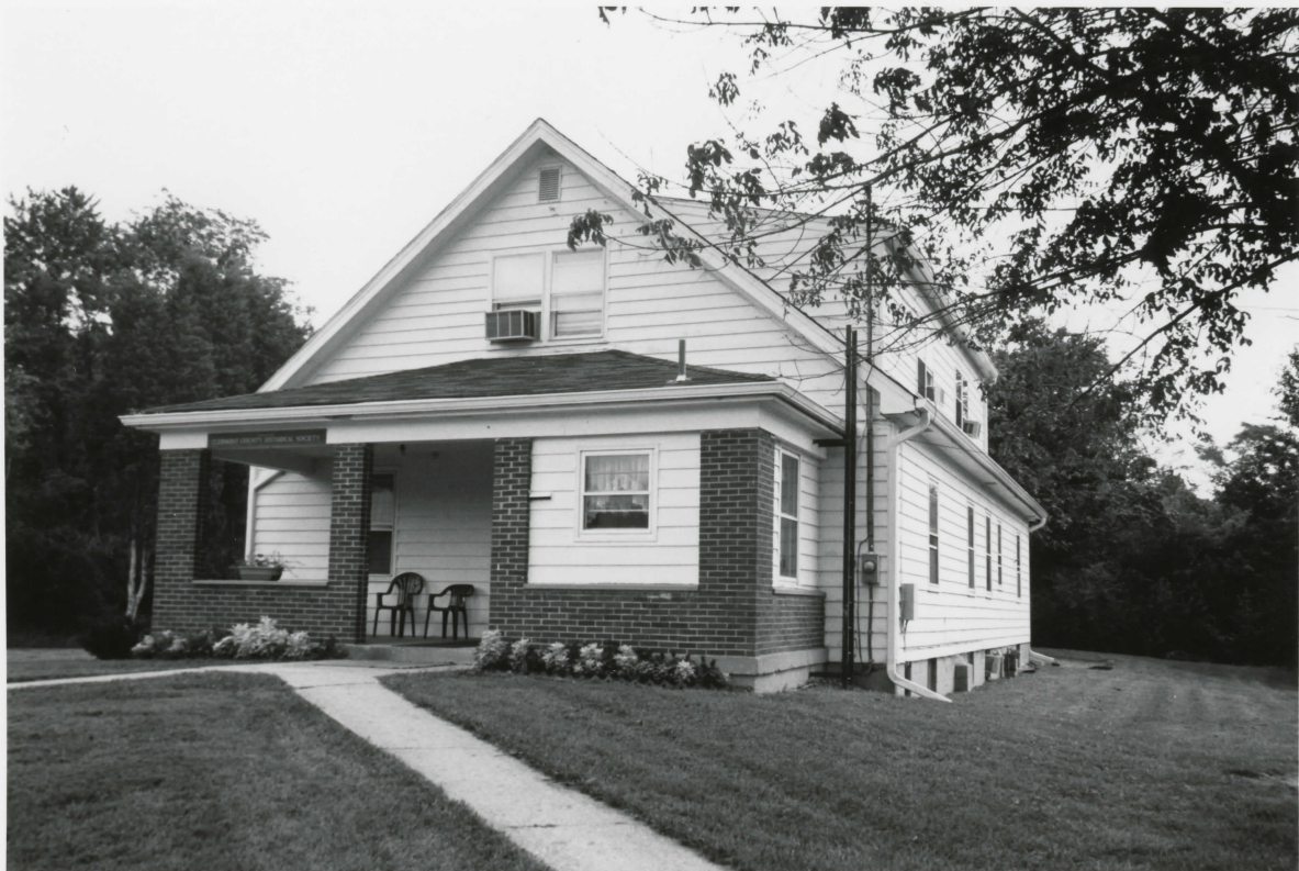
Harmony Hill Dairy House, Clermont Co., OH Photo 8
