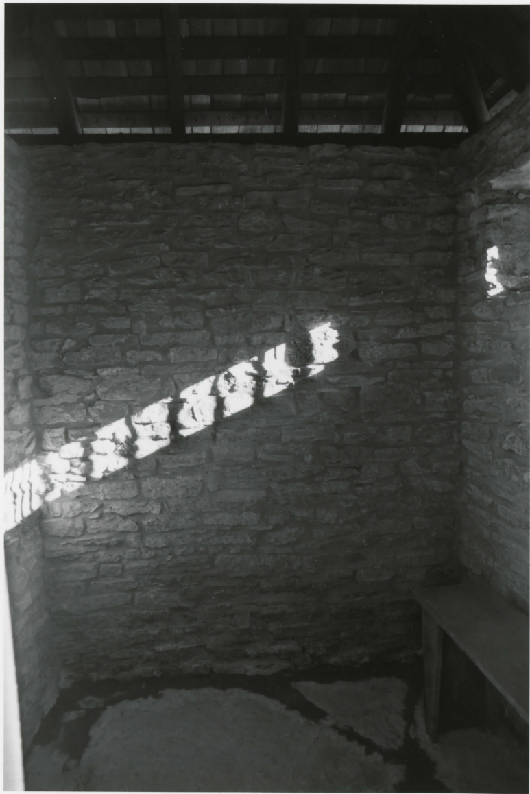
Harmony Hill Dairy House, Clermont Co., OH Photo 6
