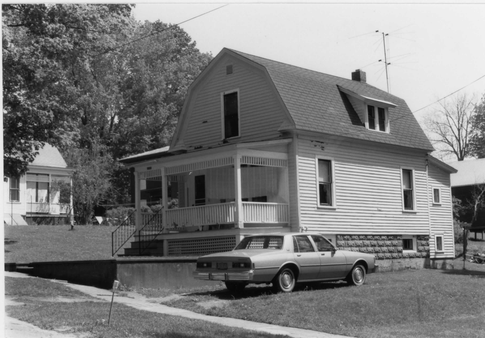
Secondary residence to the west of the house.
