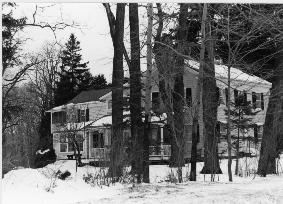
3. South elevation; looking northwest
