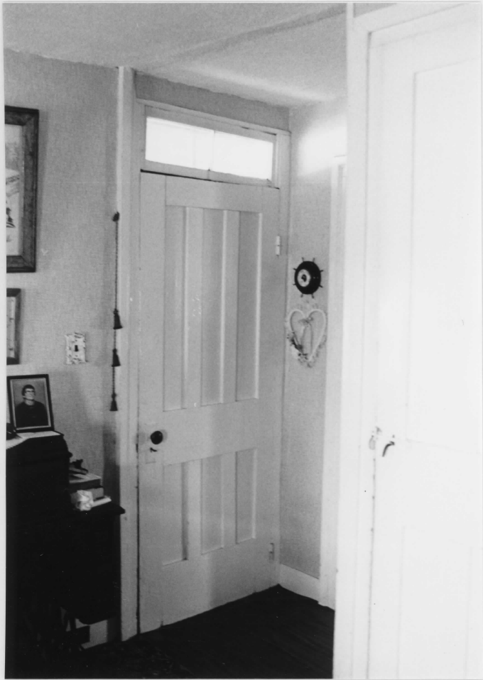
6. Door detail, front entrance
