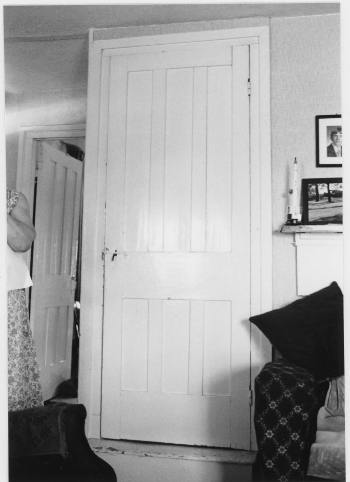
7. Door detail, entrance to staircase
