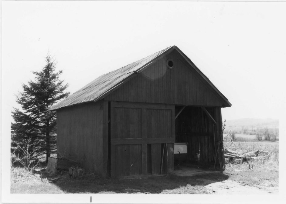
4. Machine shed; viewed from northwest
