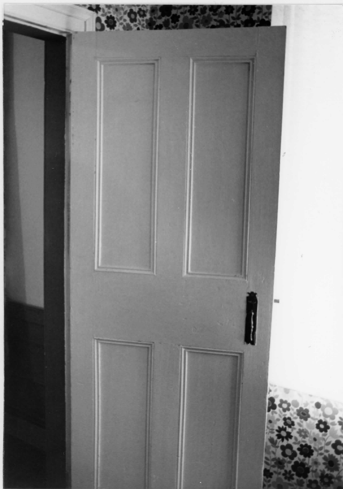
8. Door detail, upstairs bedroom
