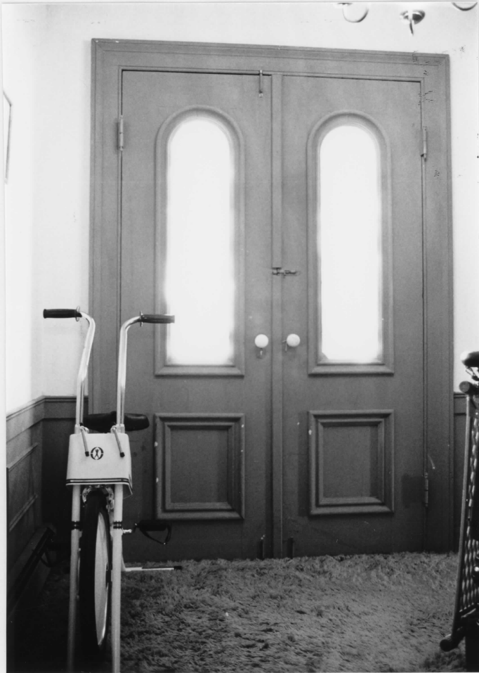
6. Detail, front door
