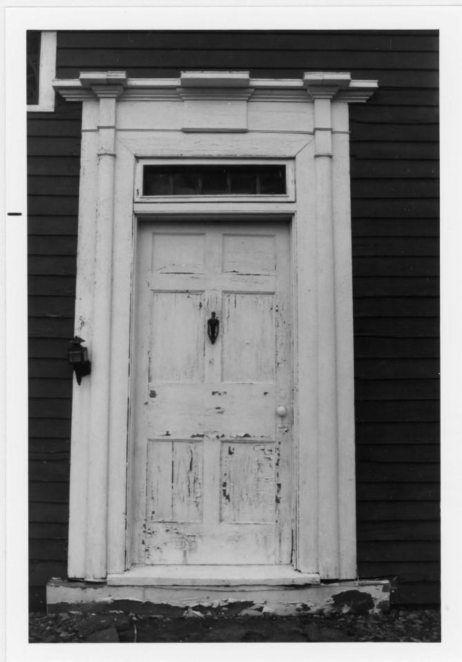
2. Main entrance; door detail
