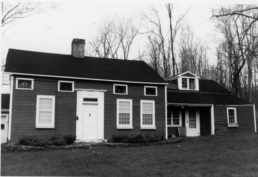
1. South (front) facade
