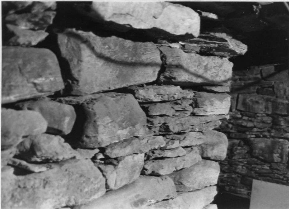
6. Basement, dry-laid stone chimney foundation
