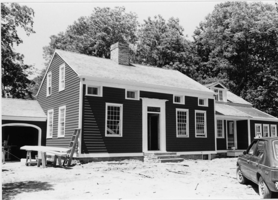
9. Restoration in progress, 1987
