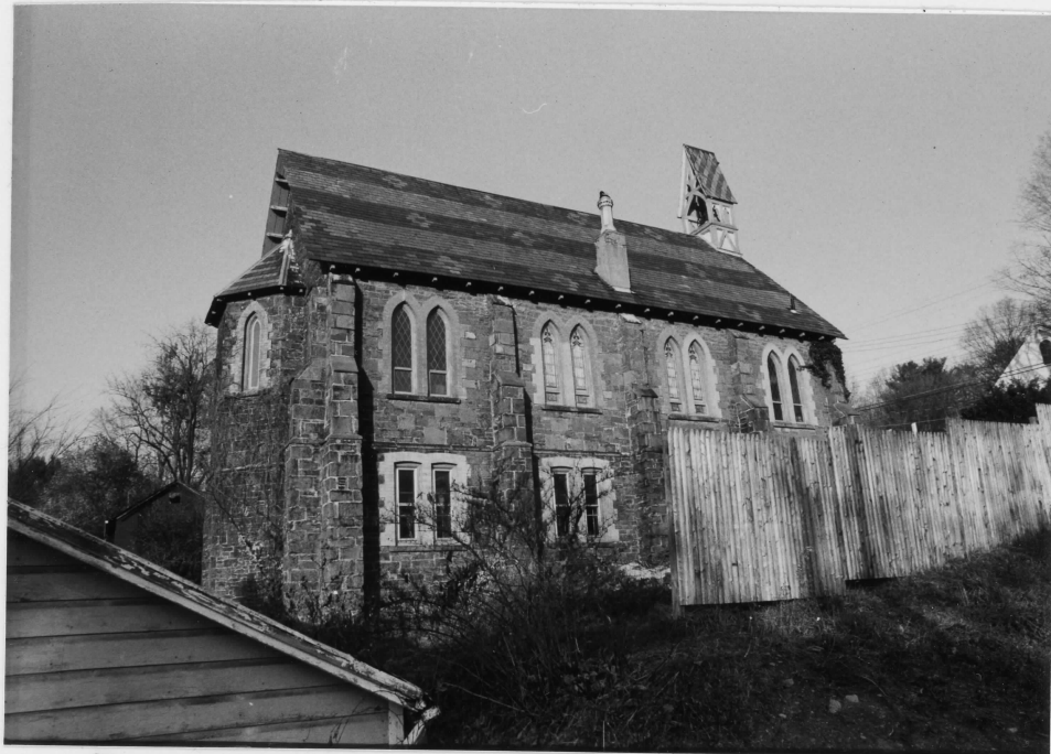
3. West (rear) and south elevations
