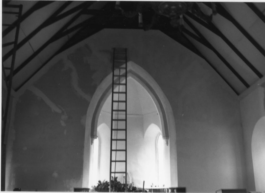
Apse, west wall
