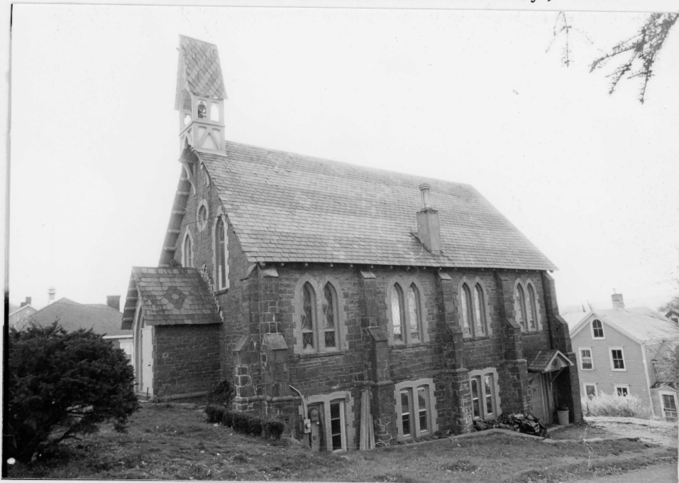
1. East (front) and north (side) elevations
