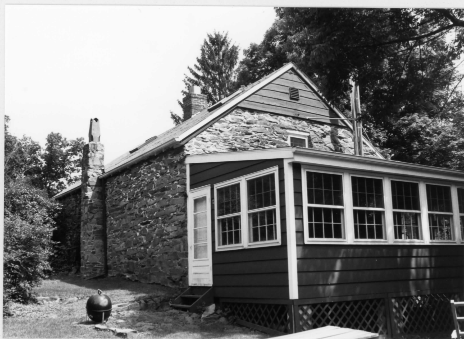
3 North and west (rear) elevations
