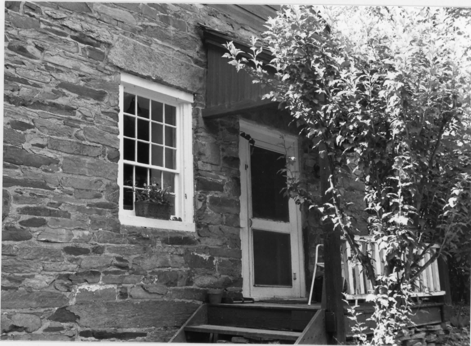
4 East (front) facade, door detail
