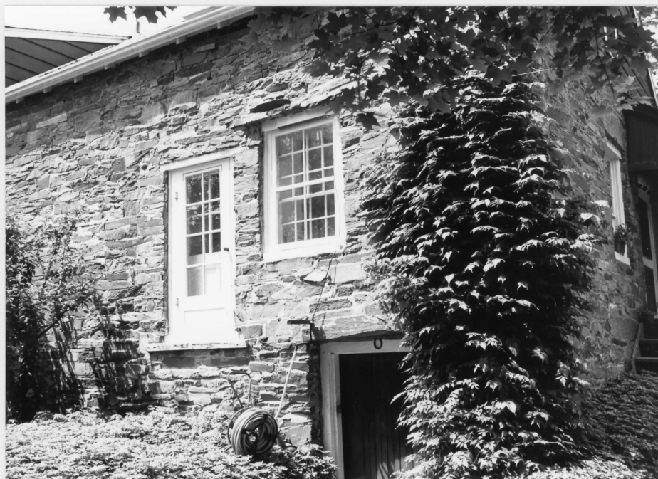
5 South elevation, door and window details
