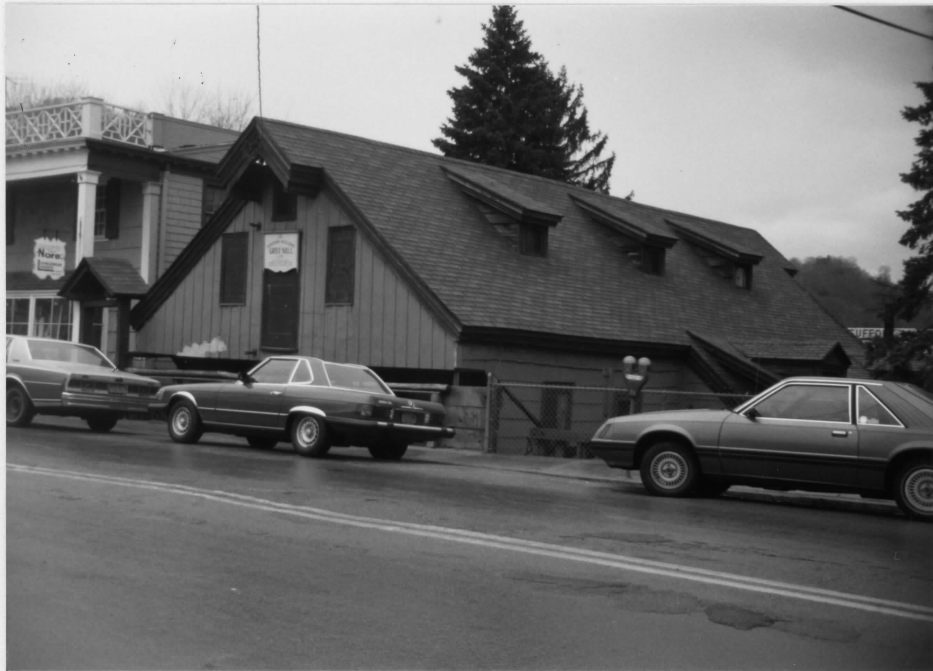
South front of mill viewed northwest from Old Northern Boulevard.
