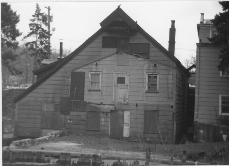
North end of mill viewed from bulkhead north of mill.
