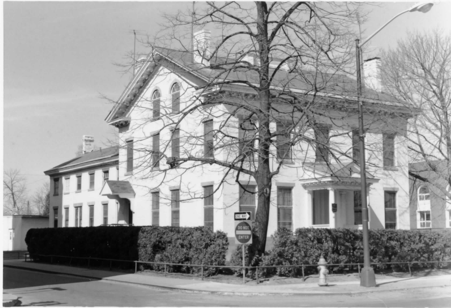
WEST AND SOUTH SIDES, LOOKING NORTH
