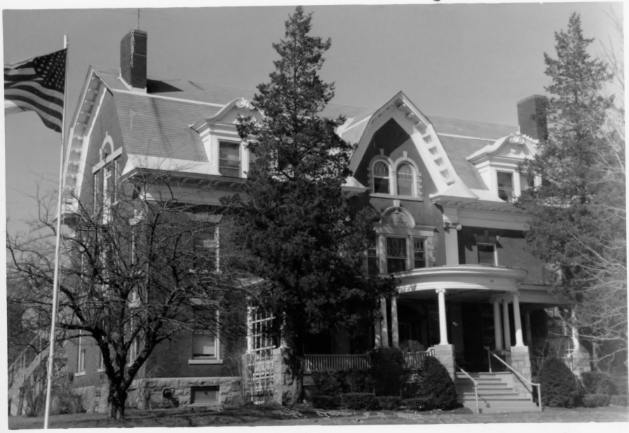
MA 7.15 SOUTH EASTERN, LOOKING NORTH
