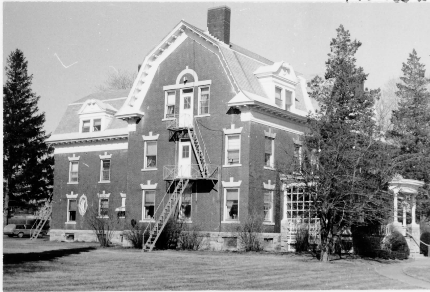
WEST SIDE, LOOKING NORTHEAST
