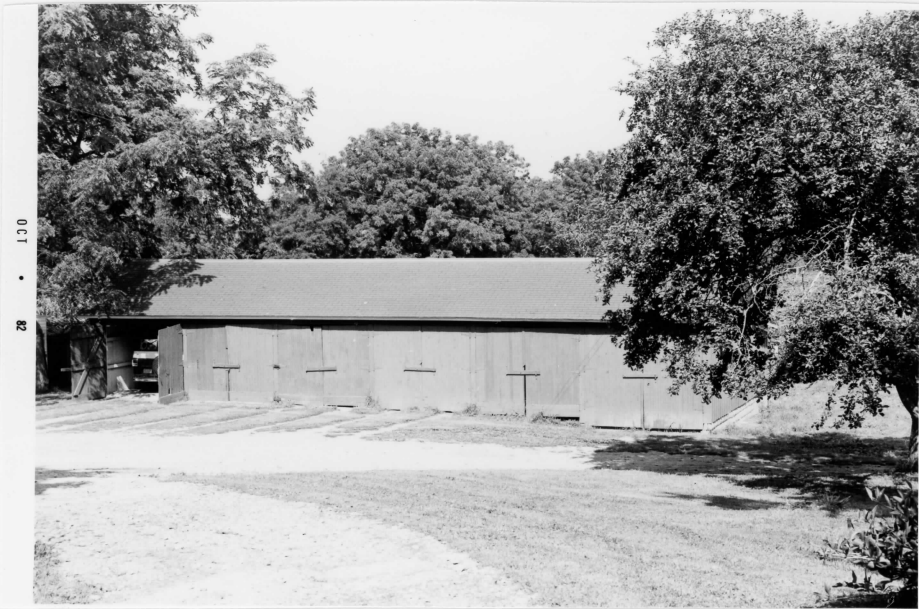
Equipment Shed View from southeast
