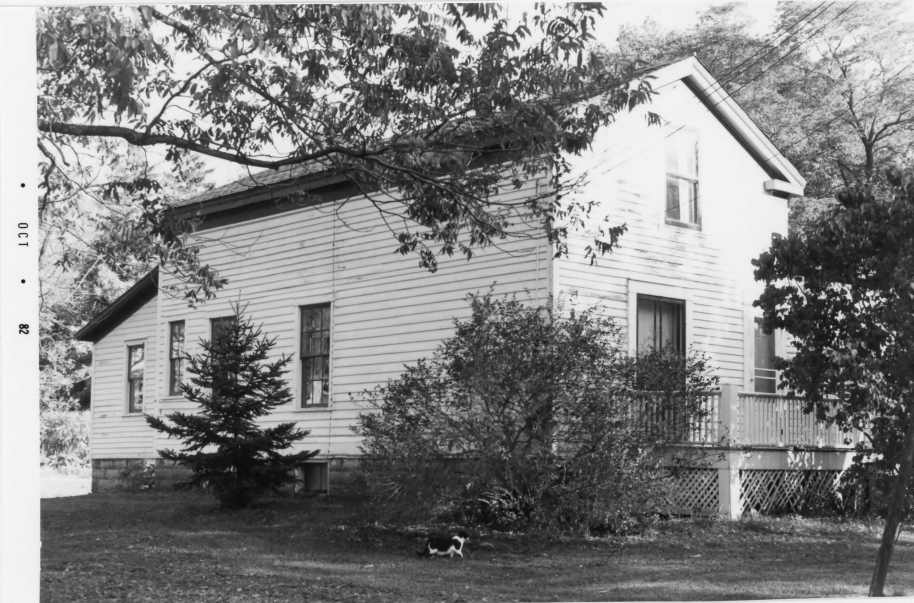
Tenant House 17 Persons Street Non-contributing
