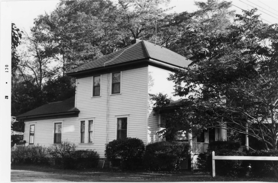
Tenant House 15 Persons Street Non-contributing
