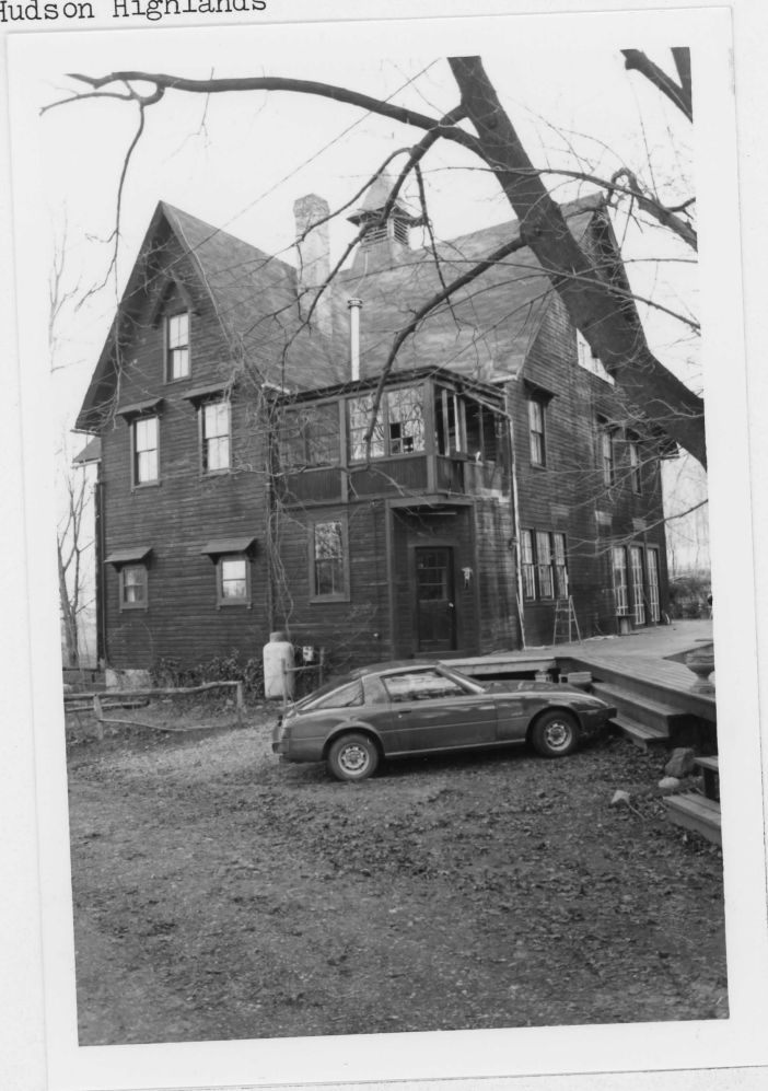
View of the Carriage House from the southwest
