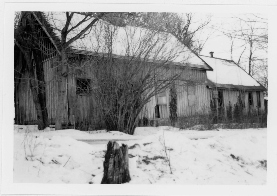
North facade of cow barn
