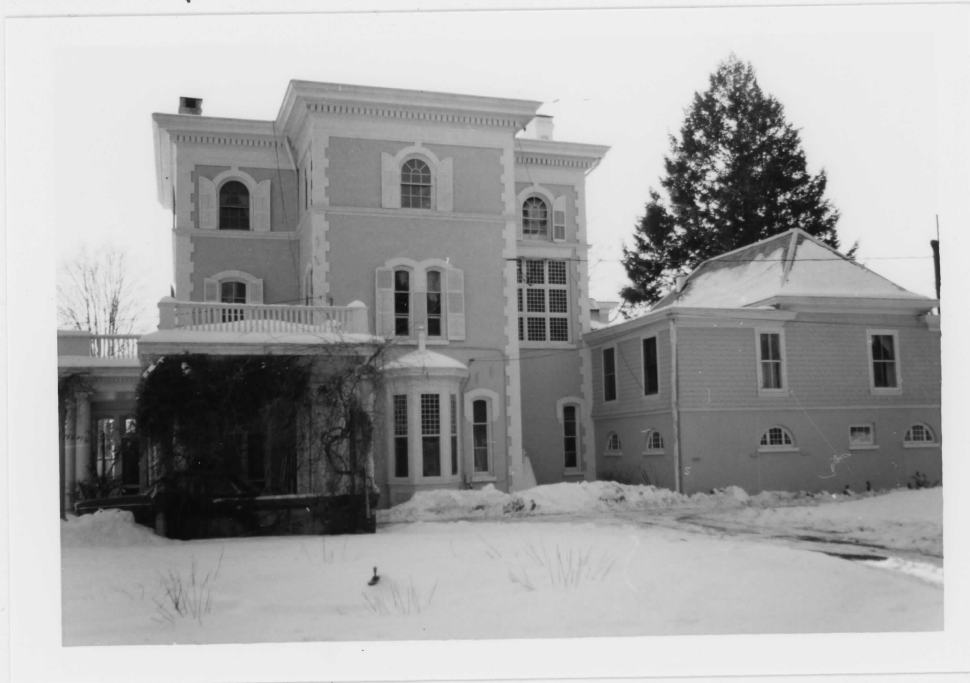
East facade of Fair Lawn
