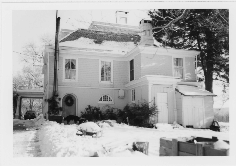
North wing and addition
