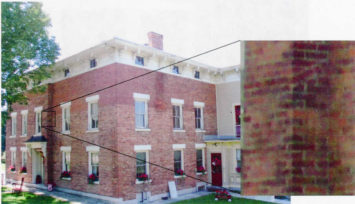
Detail of west elevation with arrow showing remnants of wooden frieze band (above) View of main elevation and wing with detail of angled bricks showing former roofline.
