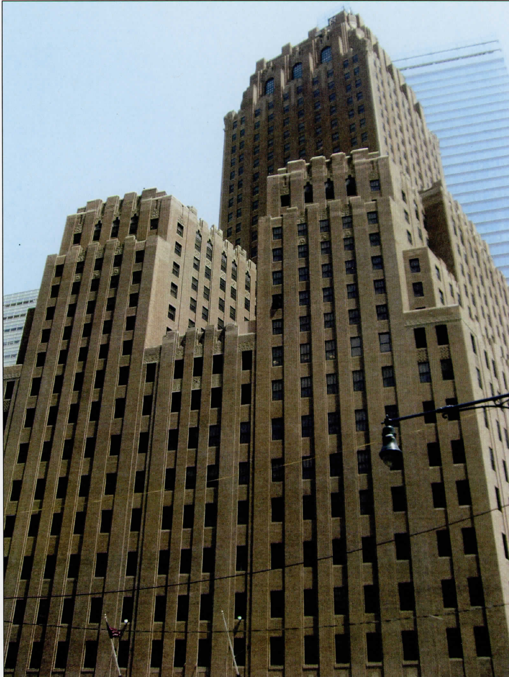
Figure 2: Barclay-Vesey Building, West Elevation (floors 3-32)
