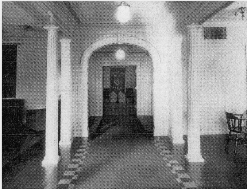
Entrance foyer, 1920s historic view
