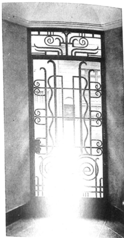
Fig. 71 A large Monel Metal grille, 42" x 60", designed by Henry Allen, Inc., Architects, New York City, and installed in the entrance to the New York Public Library.
