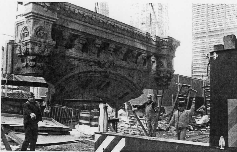
Installation of north entry arch (below)
