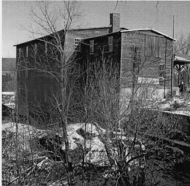
West (L.) and South elevations from Bear Gulch, view North
