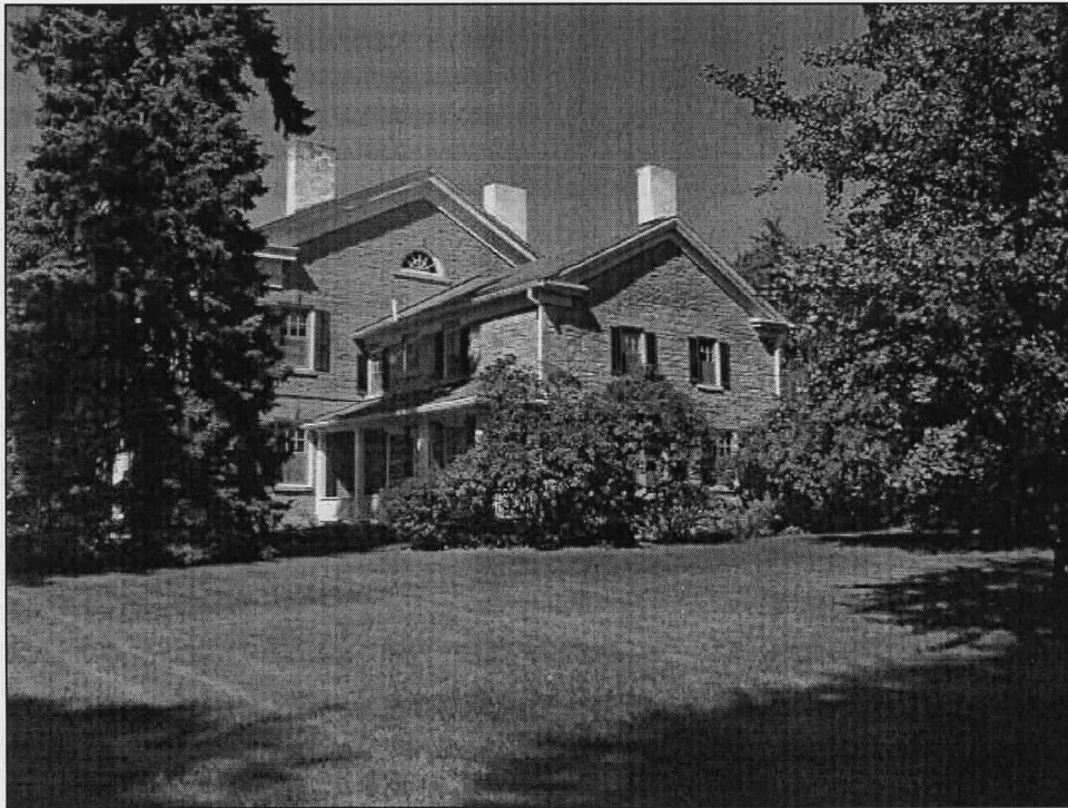
Front (south) and side (east) of 1792 kitchen wing and east end of 1816 main block
