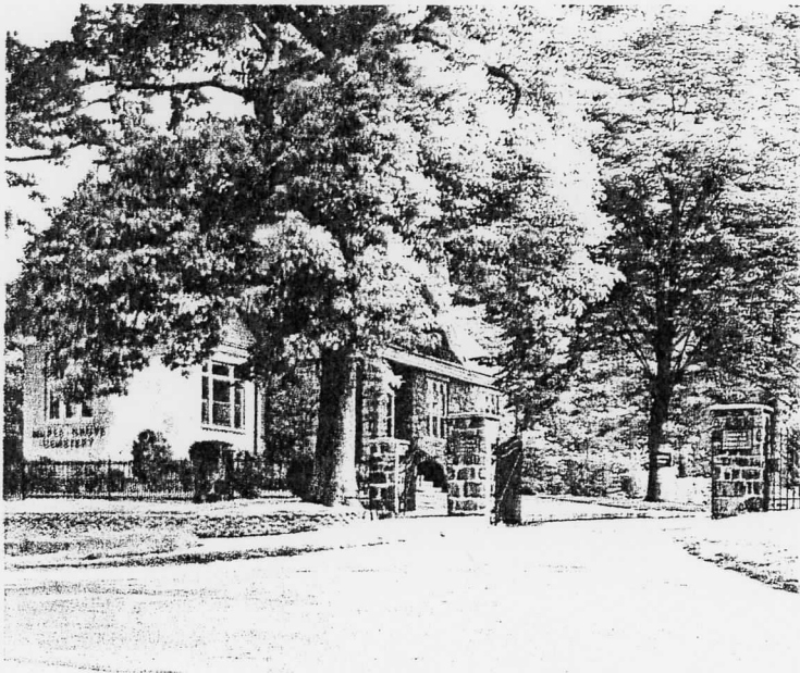
Gates at Administration Office.
