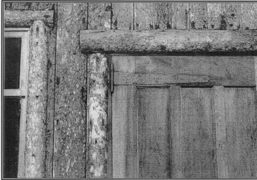
Detail of door and window trim and bark-covered siding
