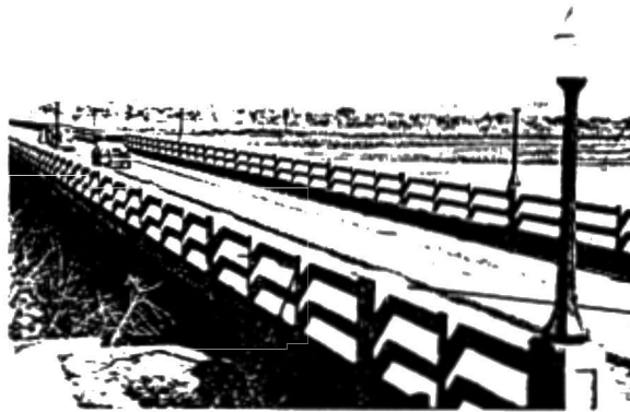
Barelvas Bridge Across the Rio Grande at Albuquerque. Completed in 1928, the Barelvas Bridge included timber pilings, steel floor beams and a concrete deck. (Highway Department Bridge Files, Inactive)
