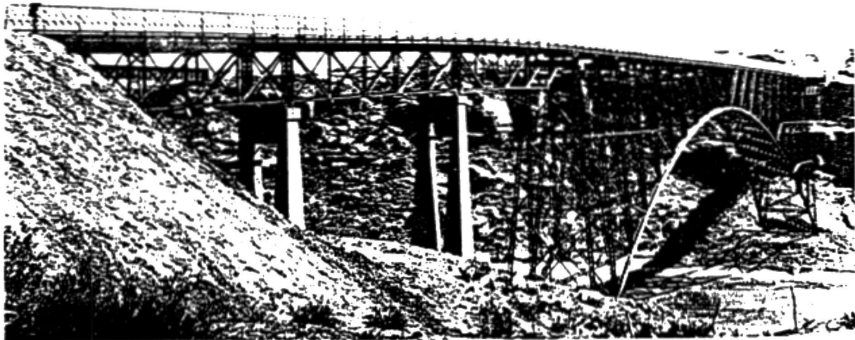
Canadian River Bridge at Logan. This steel arch bridge was completed in 1922 as an early Federal-Aid Project. (Highway Department Bridge Files, Inactive)
