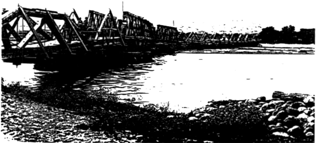
Timber Truss Across the Rio Grande at Espanola About 1912. (Photograph Courtesy of the Museum of New Mexico. Negative No. 61684)
