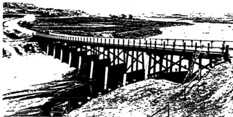
Revuelto Creek Bridge East of Tucum- cari. This bridge was completed on US 66 in 1931 using treated tim- ber construction. (High- way Department Bridge Files, Inactive)
