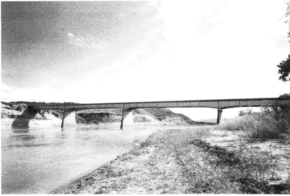
Photo 0001. Fred Robinson Bridge. West elevation. View to the east.
