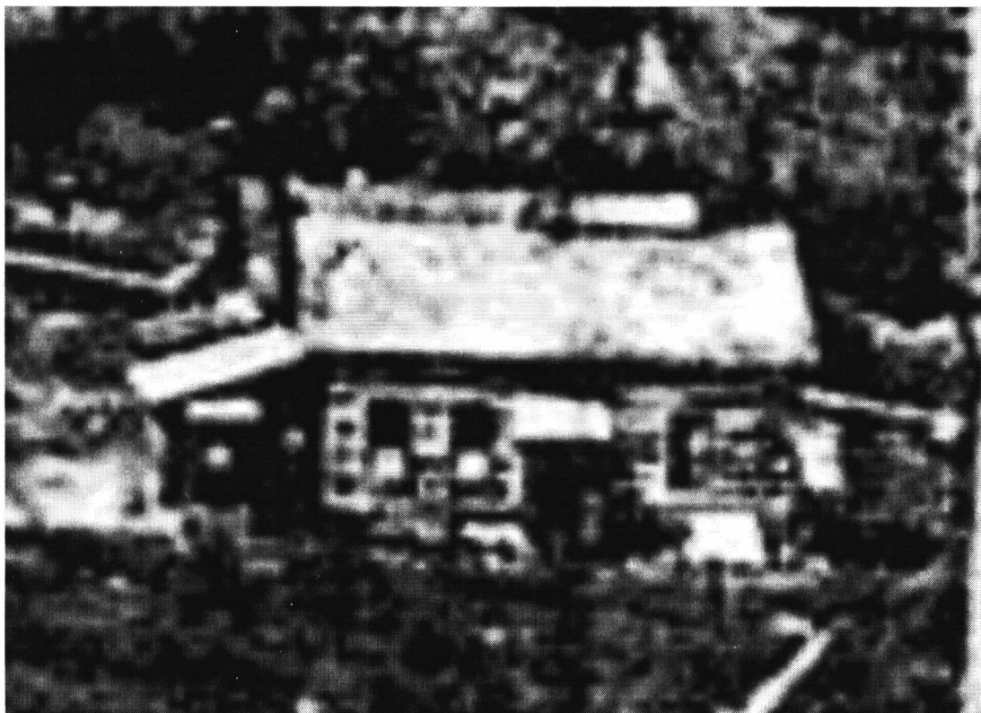
Enlarged, cropped detail from early 20 th century panorama of Lion and Cleve Mountains. Photo shows the Hecla Residence. Note the shed roof above the entrance and the lean-to at the west side of the building.
