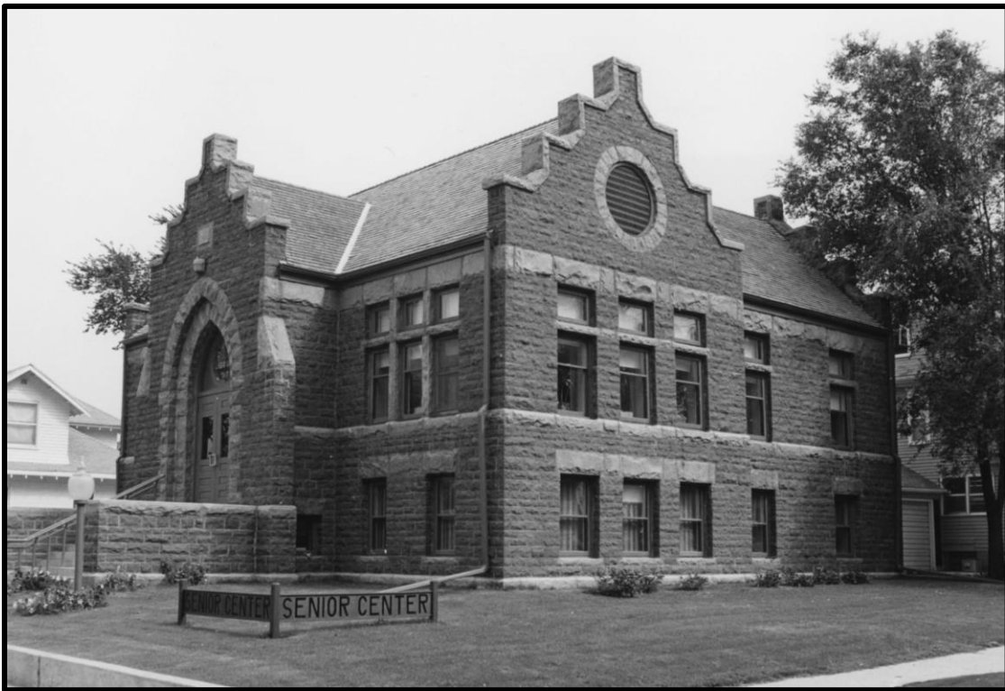
Pipestone Public Library, Pipestone County MRA, 80002122
