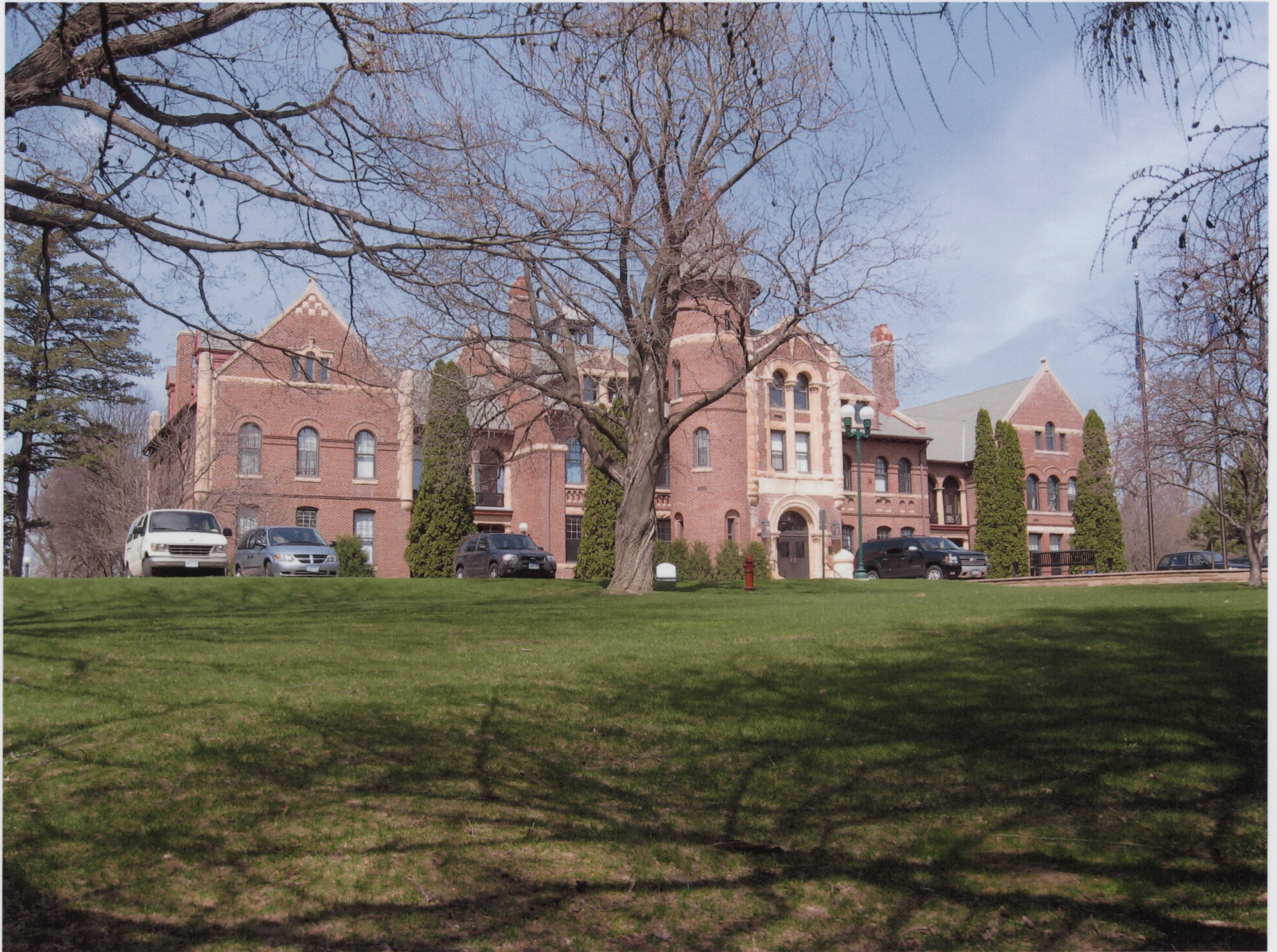
MN SteeleCounty MNStatePublicSchoolHistoricDistrict AdministrationBldg 0001
